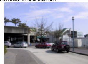
SeaBus passenger pick-up & drop-off area McDonalds in SE corner.
