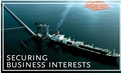
Oil Pipelines & Facilities
