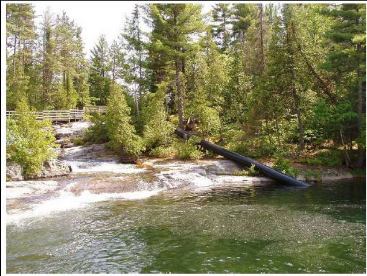
Micro Hydroelectric Generation
